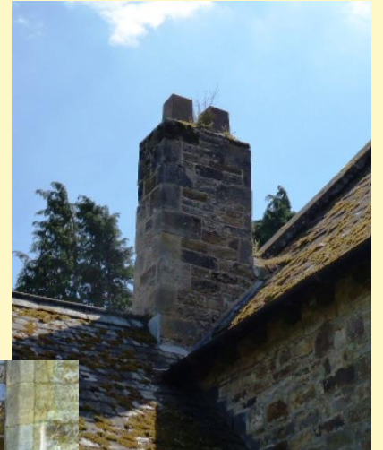
Sapling at top of chimney, defective joints in stonework
